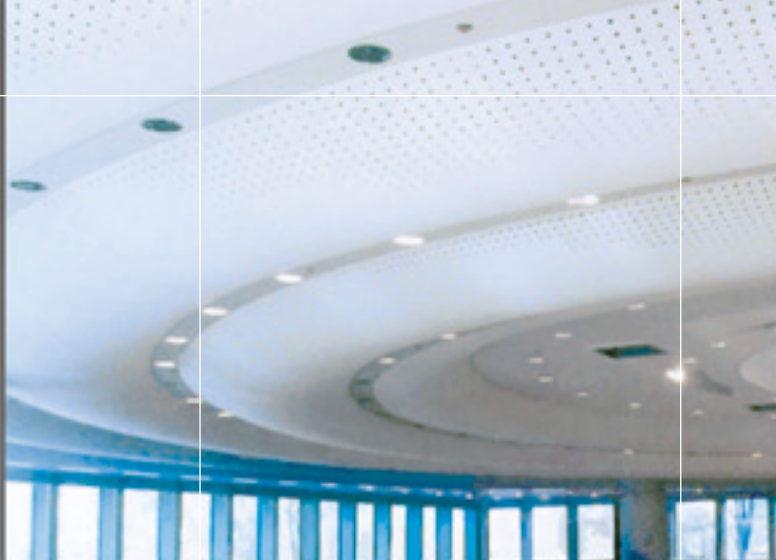
PEPSICO, PURCHASE, N.Y. Design: Gwathmey - Siegel & Assoc. Double curved perforated elements, with taped joints to achieve a continuous look.
