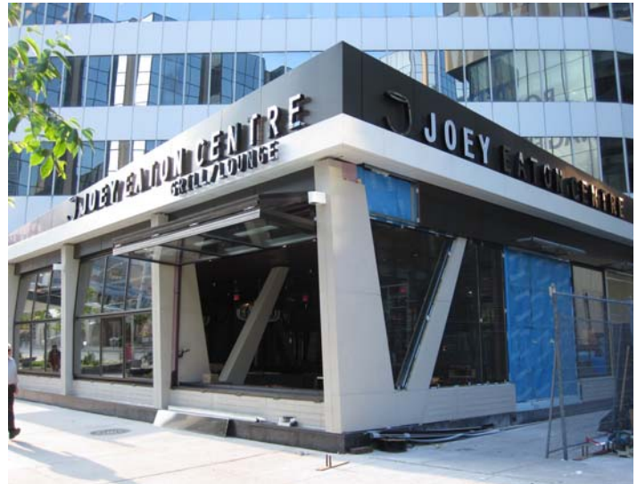
"Wishbone" Column Cladding Joey Restaurant, Toronto (Photo shows installation in progress)
