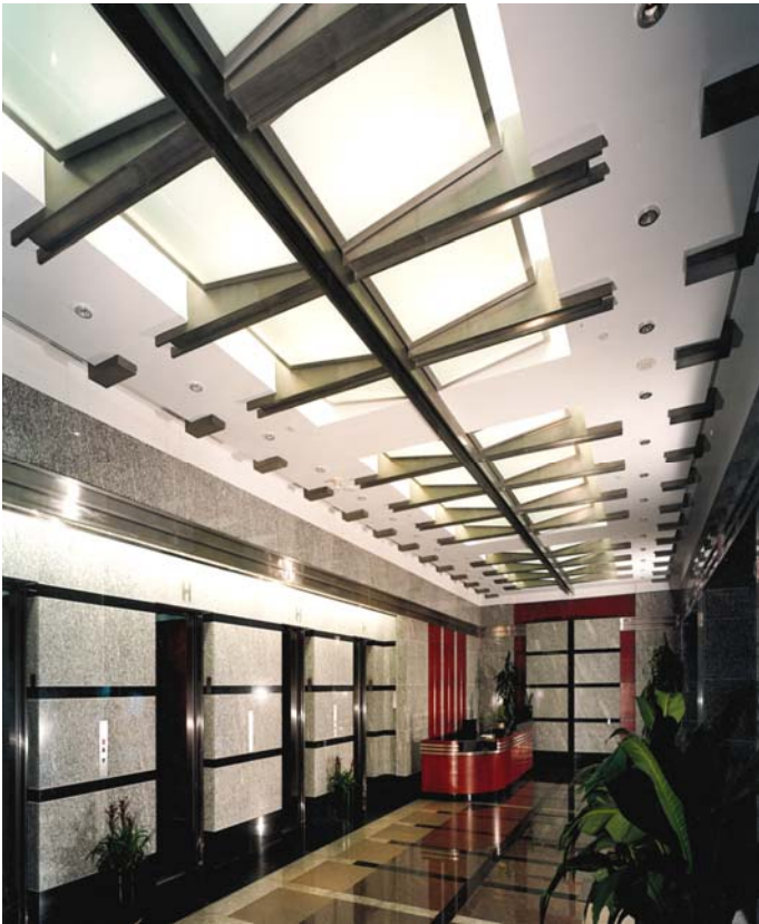
Ceiling Beams and Brackets 1775 Eye St. Washington, DC
