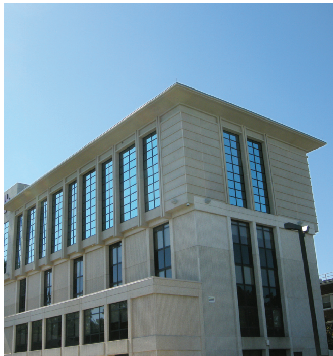
WINDOW MULLIONS AND CLADDING PANELS
