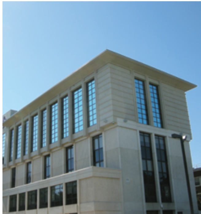
WINDOW MULLIONS AND CLADDING PANELS
