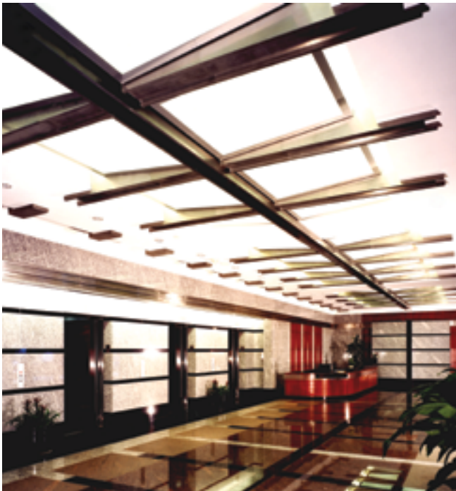
CEILING BEAMS AND BRACKETS
